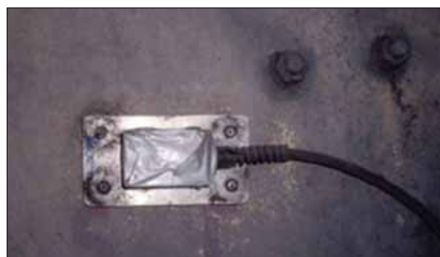
Accelerometers attached using magnets to the screen side plates.
